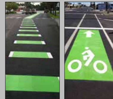
White symbols must be retroreflective. A PreMark® Bike Panel integrates easily at specified intervals while maintaining pleasing color consistency.
